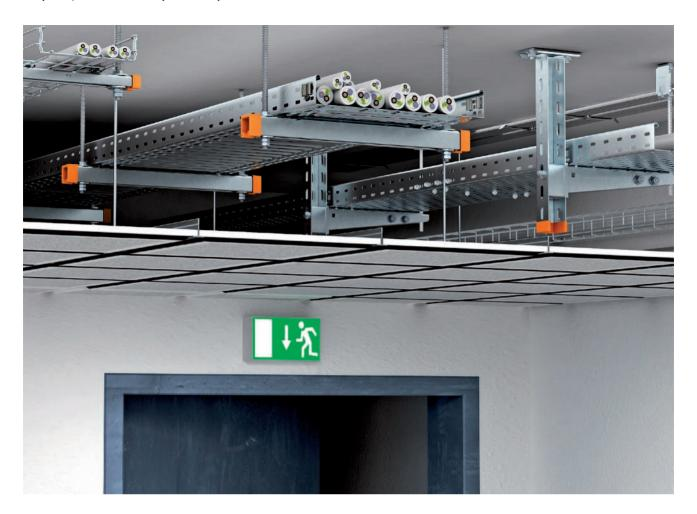
There is no testing standard for installations above fire protection ceilings and thus no classification is possible. Test criteria are the deformation of the support systems, as well as possible falling due to heat. The tests need not be carried out by an accredited testing institute but can, in principle, be carried out and documented by the manufacturer themselves.
