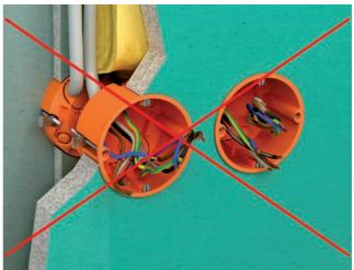
Use of special fire protection cavity wall sockets, installed on the other side next to doors with fire resistance.
