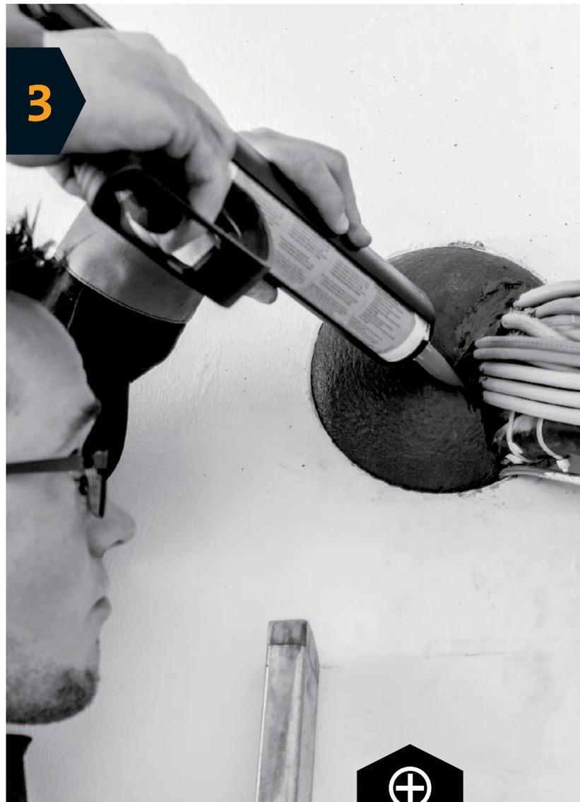
The installation engineer cuts the plugs according to the cable assignment. Then they are pressed into the wall opening quickly and cleanly on both sides - without dust or fibres. Installation must always take place according to the approval.
